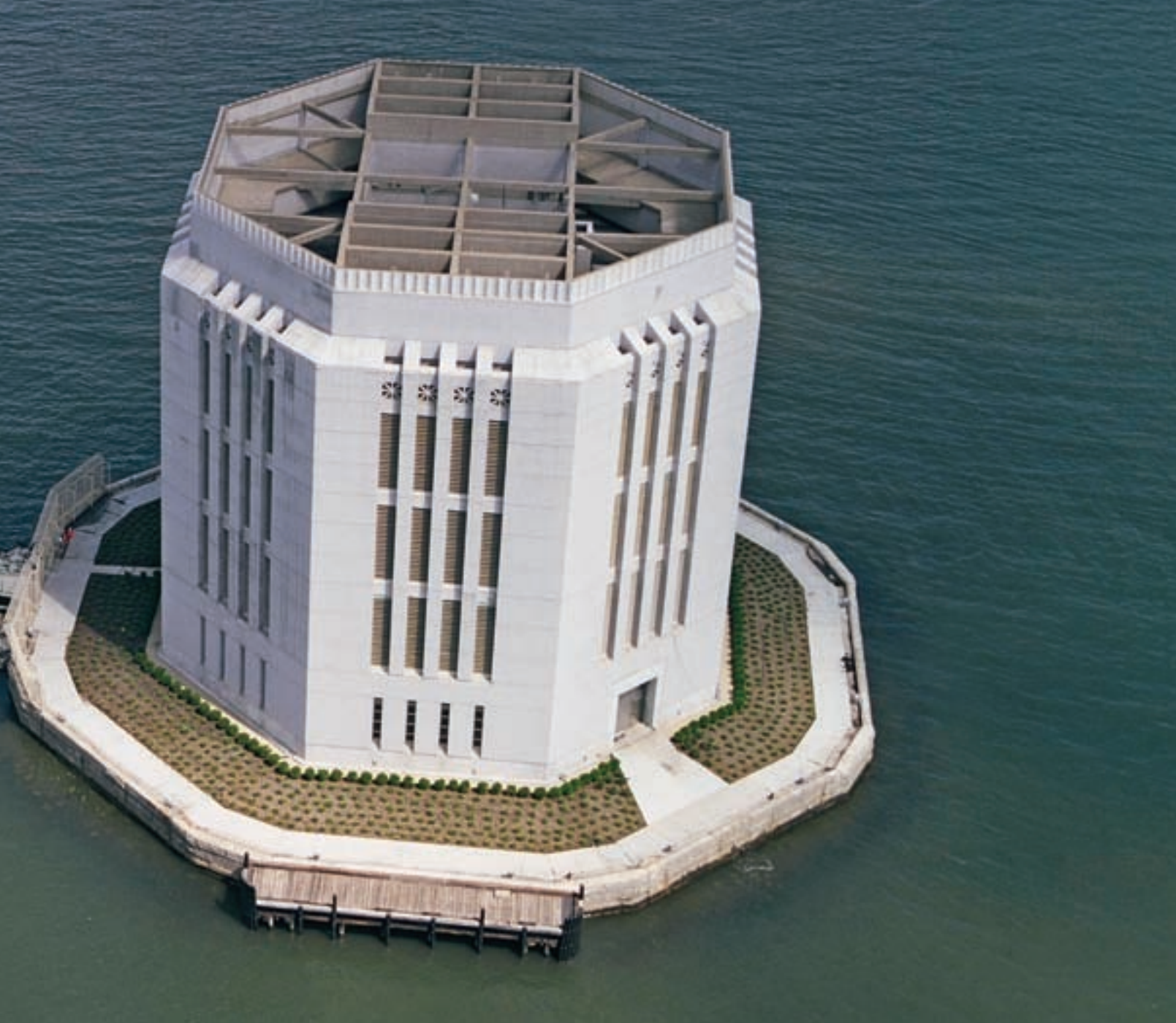
ABOVE: Aerial view of the exterior of MTA TBTA Brooklyn Battery Tunnel Governors Island Ventilation Building after renovation.
