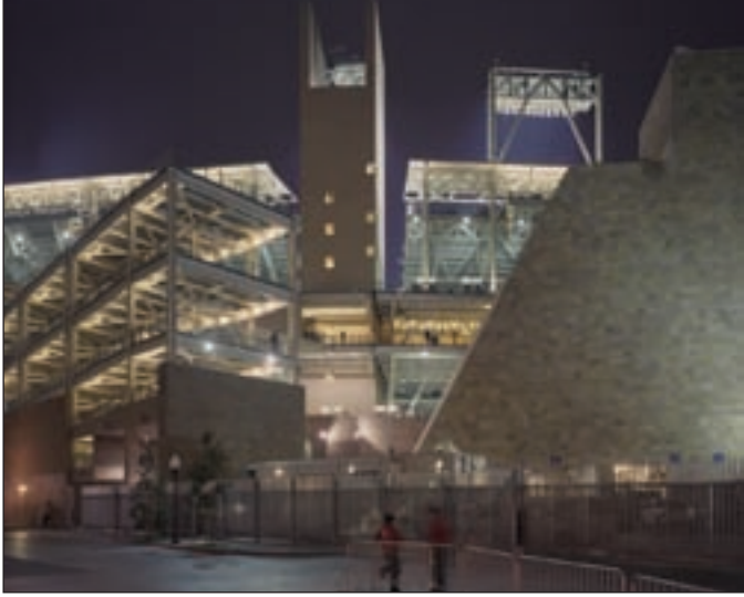
TOP LEFT: Night view of lighting tower and Third Base Building.
