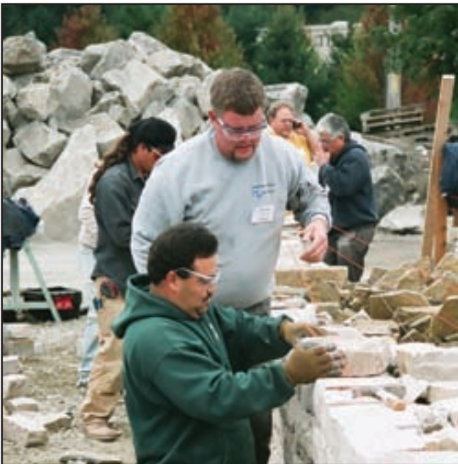
CLOCKWISE FROM TOP LEFT: Photo 1: Drystone bridge in progress.
